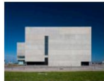
Fachada lateral norte- foto: Archdalaly
